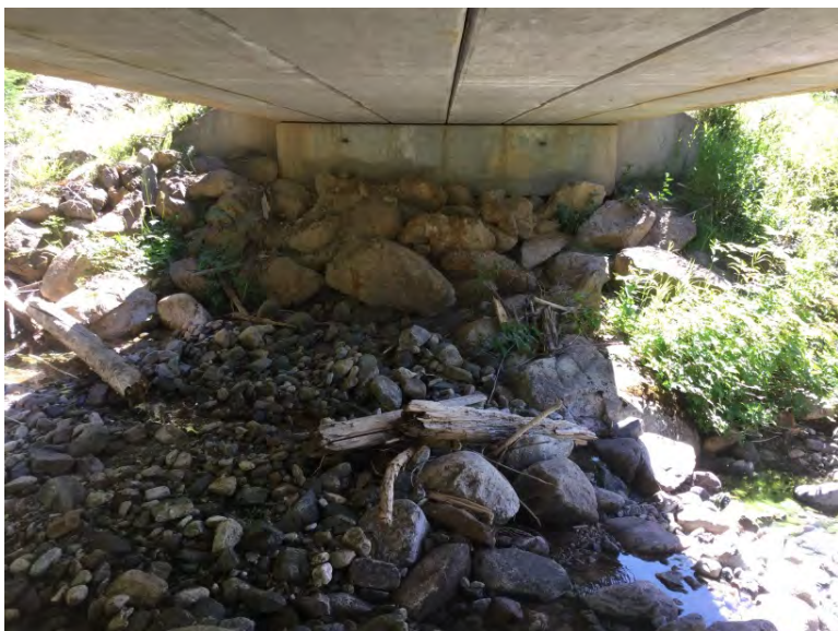
Left Bank Abutment when facing downstream
