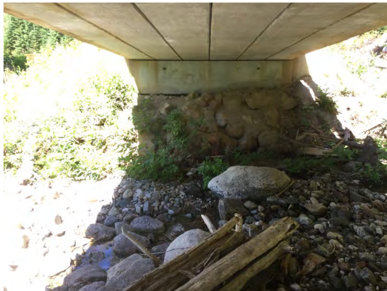
Right Bank Abutment when facing downstream
